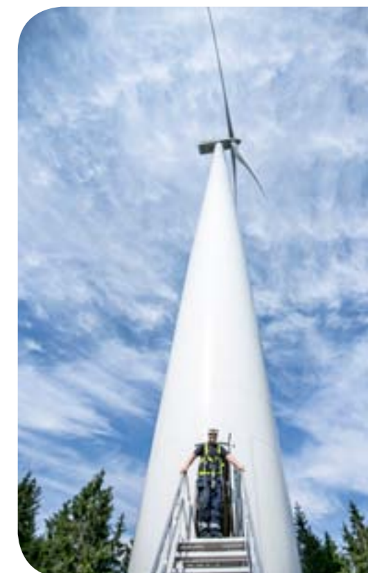
Vindpark Hakarp, Ronneby
